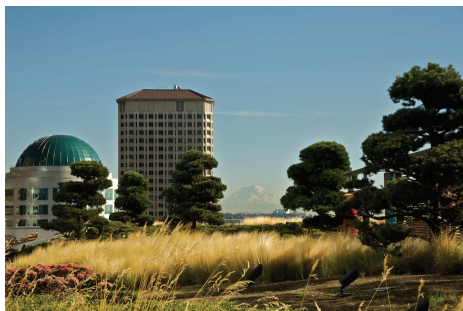
Green roofs aid stormwater management
