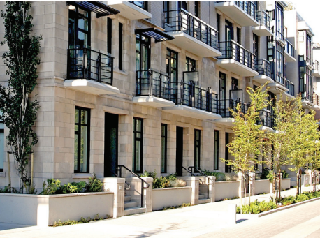
Street facing front entries with small terraces, entry stairs, a slightly raised first floor, and landscaping.
