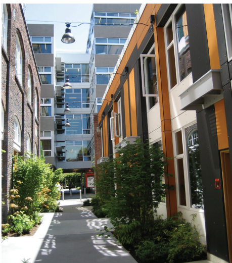
Changes in materials and textures combined with sizeable recesses and alterations in building height create visual massing breaks.
